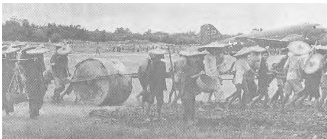
This is just a small insight into the amount of human labor that was necessary to build the airfield in the India-China Command. Earth was moved in the same fashion as it had been for thousands of years. Also, note rollers pulled by crew.
